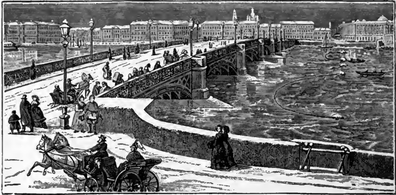
THE NICOLAI BRIDGE, ST. PETERSBURG
